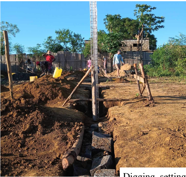
Digging, setting, and pouring foundation and column supports
